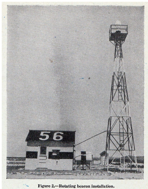
Figure 2.—Rotating beacon installation.
