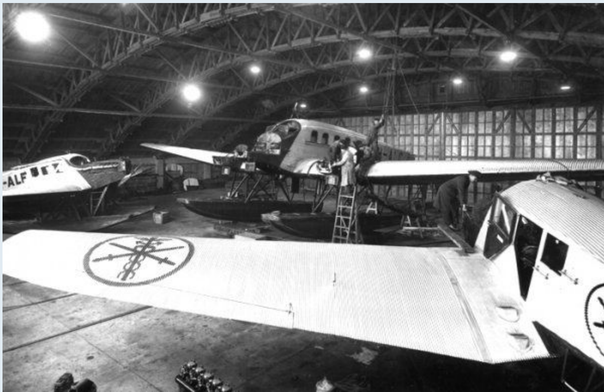
November 1st, 1932: A major overhaul of the Aero Oy Junkers G-24 in progress in a workshop adjacent to Aero Oy's Kellosaari Hangar. Helsinki got its land airport in 1936 when Malmi Airport was opened and at the same time Aero Oy built a modern hangar for maintenance activities
